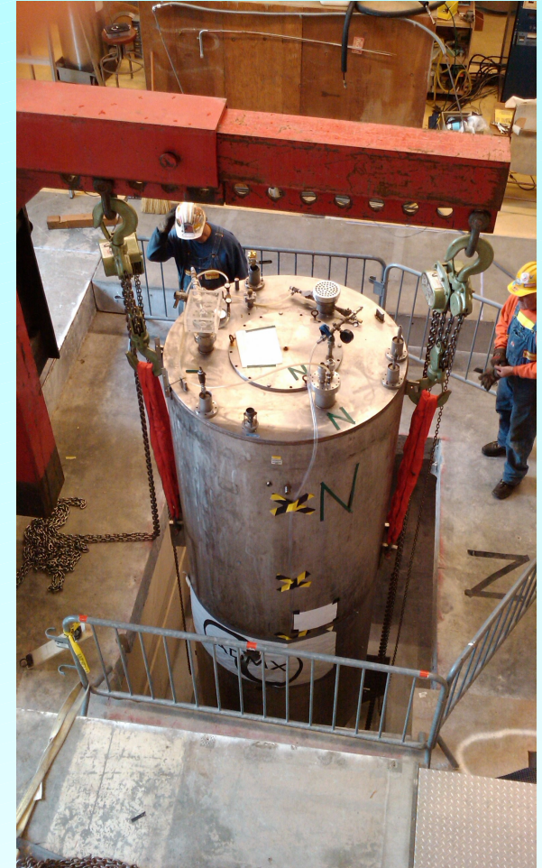
May 2011: Main Magnet Installed in Experiment Area (CENPA)
